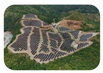
This global collaboration—drawing expertise from Malaysia, Japan, Germany, China, and the Philippines—launched in May 2024 and features a 29.952 MWp Double Glass Solar PV System integrated with a 4.386 MWh Battery Energy Storage System (BESS), the first of its kind in the country.
